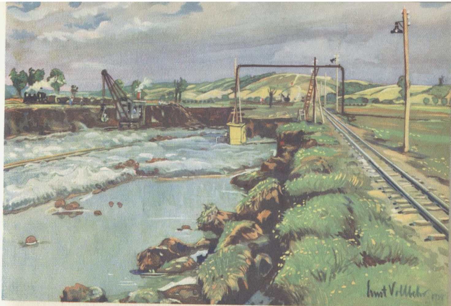
Baustelle Randowbruch, Mooraushub
